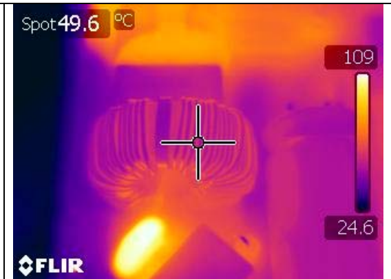
Figure 54 - Common Mode Choke (L1), 115 VAC Input, 100% Load, Room Temperature.
